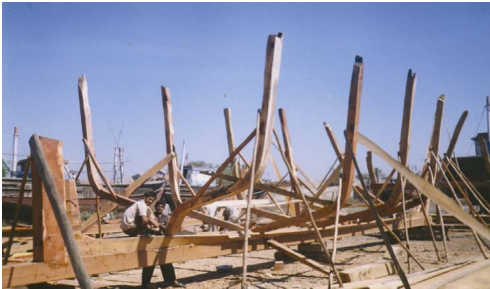
18. A traditional boat under construction
